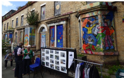
Left Houses on Cairns Street renovated by Granby Four Streets CLT, 2019
